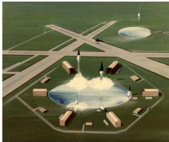
Figure 37. A Vertical Launch Complex Provides Vertical Toss Back Booster Recovery and Horizontal Landing Facilities for the Hypersonic Gliders
